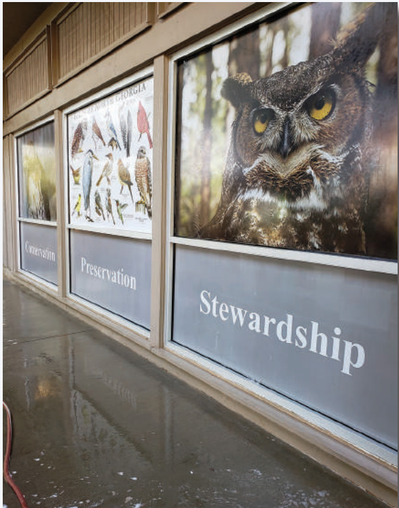
The CollidEscape films used at Sawnee Mountain show photos of Georgia birds and wildlife. The films prevent birds from flying into the windows, but are completely transparent from the inside to allow visitors a clear view of the outside. Photo by Adam Betuel.
