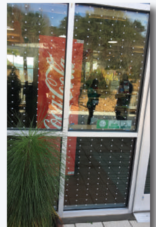
CollidEscape Film was placed on the entire Discovery Center at the Chattahoochee Nature Center using the 2017 Disney Conservation Fund Grant. The Kendeda Center at Trees Atlanta and three other buildings will be treated using the 2018 grant. Photo by Dottie Head.
